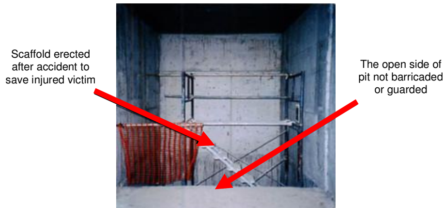
Figure 11: No barricade for pit
